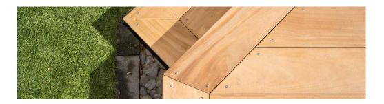
**END SEALING** will help minimize splitting and checking at the ends of the boards. We recommend the boards be end-sealed with a quality penetrating oil as soon as possible after cutting and before final installation.
